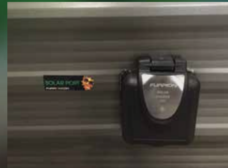
Solar Prep And Wiring
