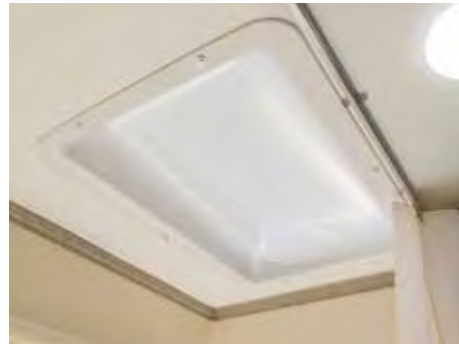
Skylight over Tub
