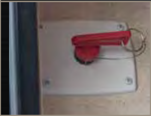
Battery disconnect in pass thru storage
