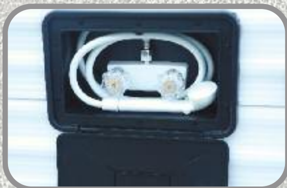
Exterior Shower with Hot and Cold Water
