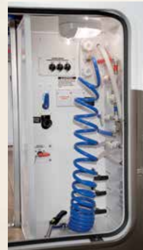
The Docking Station includes outside shower, black tank flush, water bypass, 12V battery disconnect, selector switches, dump valves, water tank and city fills for centralized convenience.
