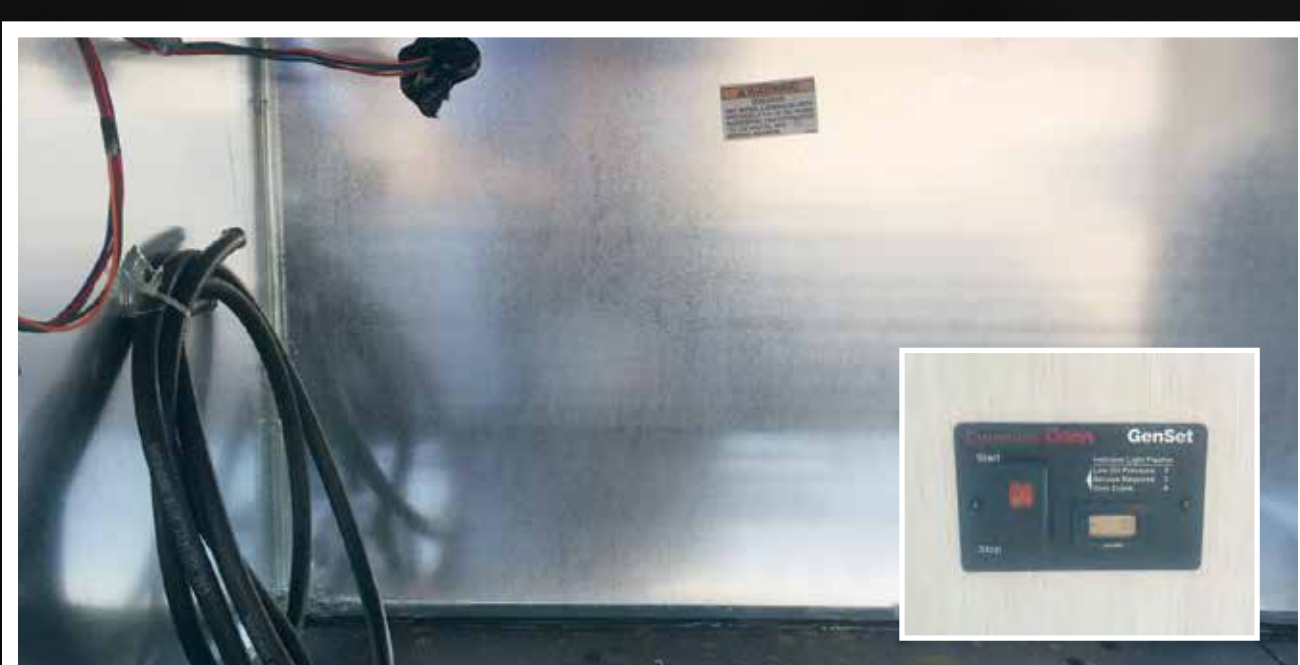
Gen Prep w/Transfer Switch
