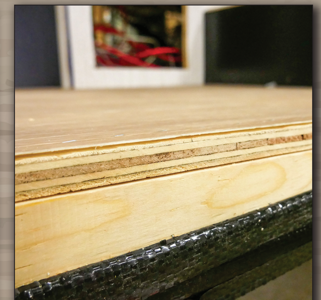
TONGUE & GROOVE PLYWOOD MAIN AND UPPER FLOORS
