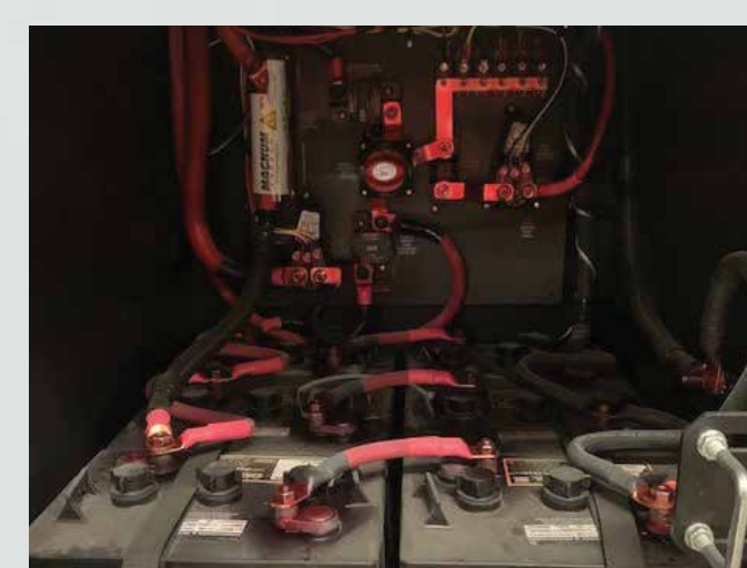
HOUSE BATTERIES (6) SIX VOLT DEEP CYCLE HOUSE BATTERIES
