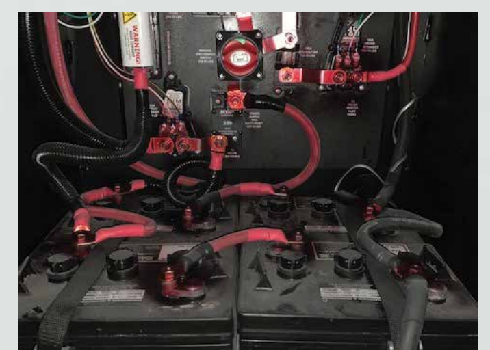
HOUSE BATTERIES (6) SIX VOLT DEEP CYCLE HOUSE BATTERIES
