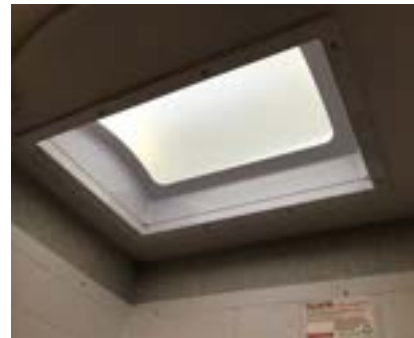
Skylight over Shower
