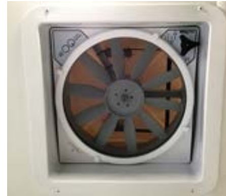
High Output Attic Fan in Bathroom
