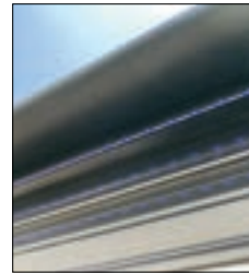
External LED Strip Lighting
