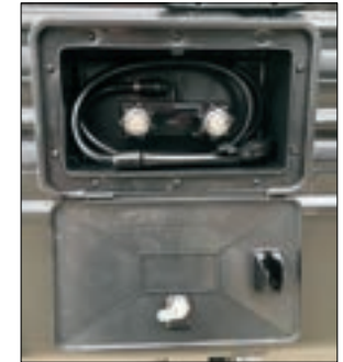
Outside Shower with Hot and Cold Water
