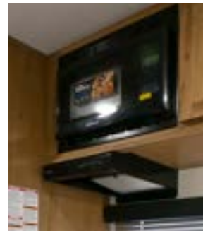
Upgraded Range Hood with Light and Fan
